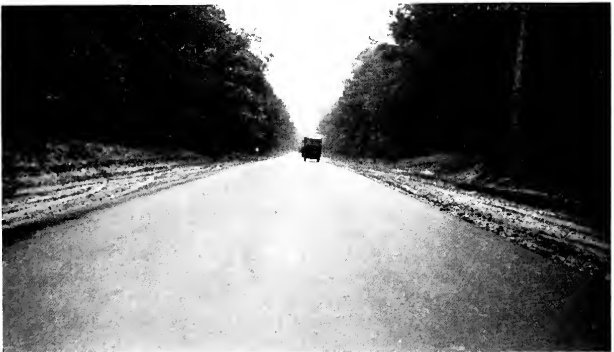
U.S. ROUTE 213—SALISBURY TO BERLIN. ASPHALTIC CONCRETE RESURFACING COMPLETED IN 1947
